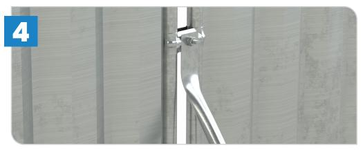
The other end of the stabiliser arm is attached to the top section of each hoarding panel using a coupler. Put the coupler in place and secure the end of the stabilizer arm using the screw and bolt. Screw the other end of the stabilizer arm down into the block tray.
